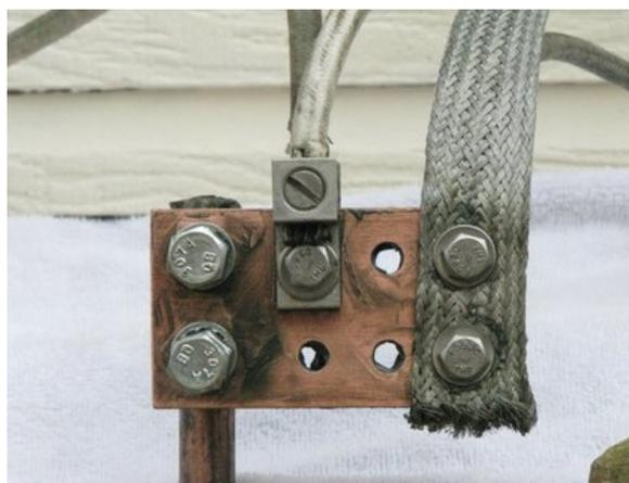
This works for me. Besides one lead from inside the shack, the others go to several other well spaced ground rods, a lead to the tower base (which has it's own ground system), and finally, the power company ground, which is only about a foot away.
